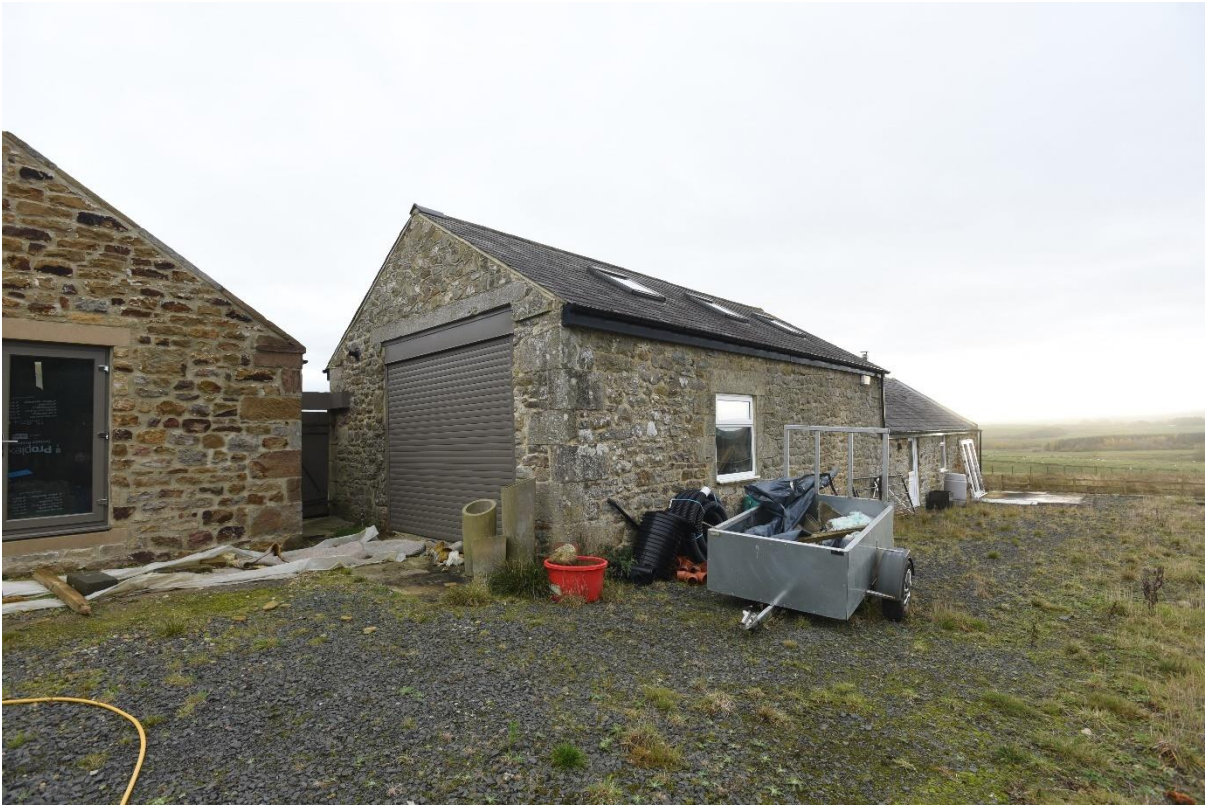
3 | Access to the workshop and boiler room on the north elevation of the annex
