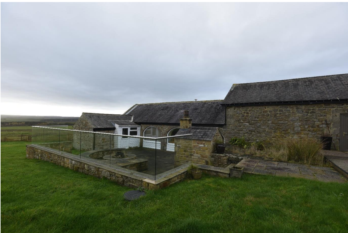
4 | Patio and amenity space to the east side of the annex
