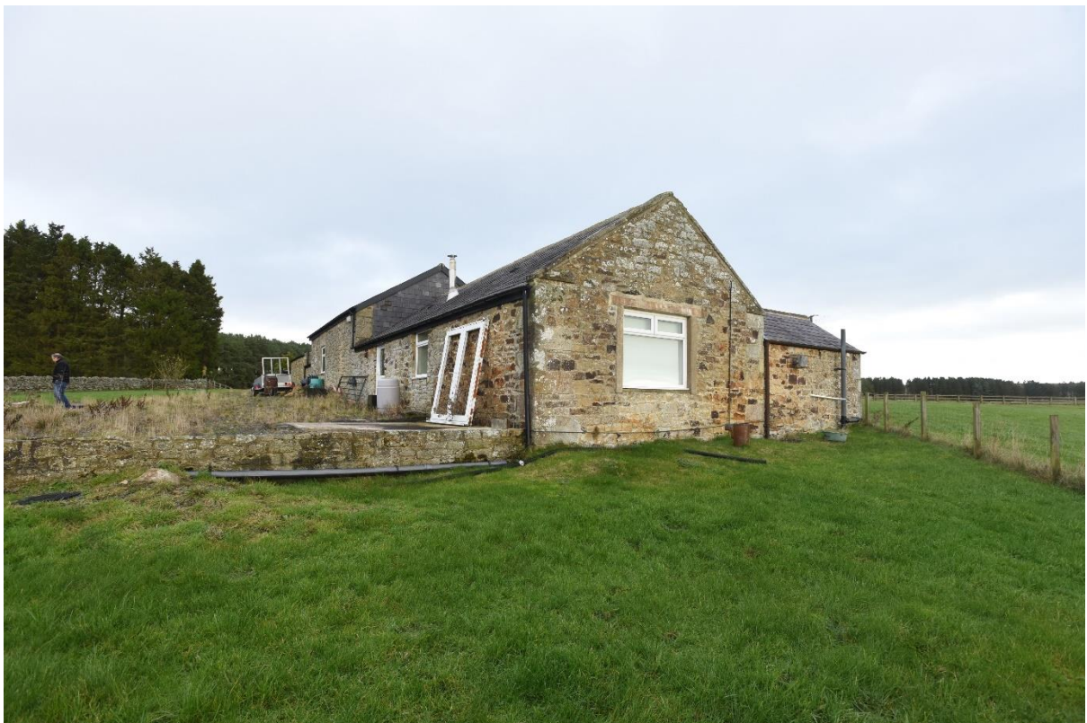
2 | Annex south and west elevations.
