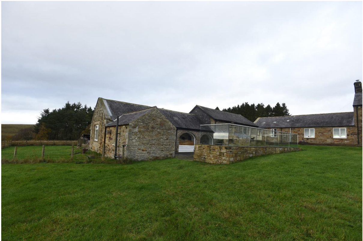
1 | Annex to the left in foreground and dwelling to the right in the background. Looking northwest from the garden
