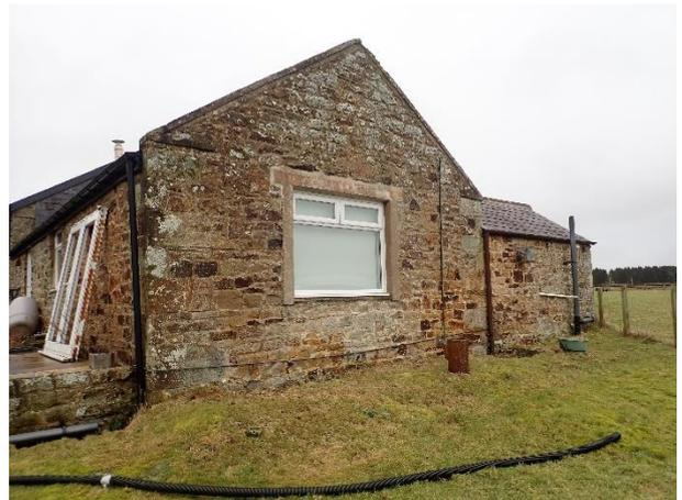
**East gable of small extension, well sealed with a sound mortar fillet.**
