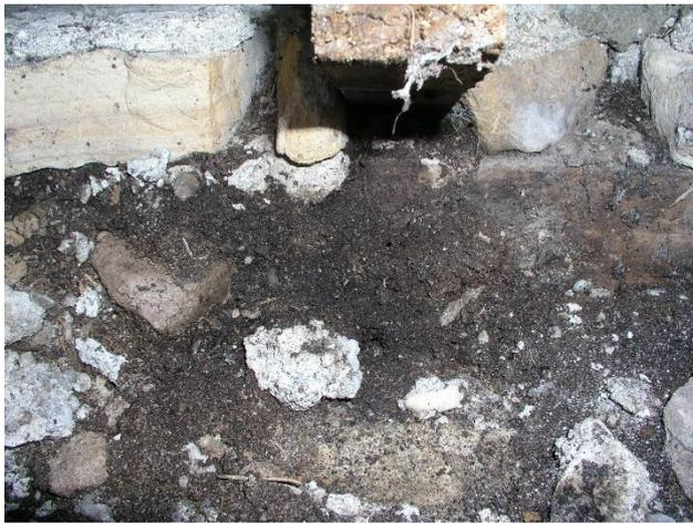
**Photo showing disintegrated bat droppings beneath coping stones. If examined carefully, in the black dust exoskeletons of insects can be seen shining.**
