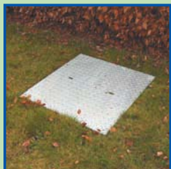
CLF1 - 6pe Fully Installed.
