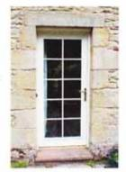
The doors would be designed to be like-for-like replacements – two would be fully-glazed with 8-panes per door whilst the other two would be half-glazed with a grooved timber panel below the mid-rail.
