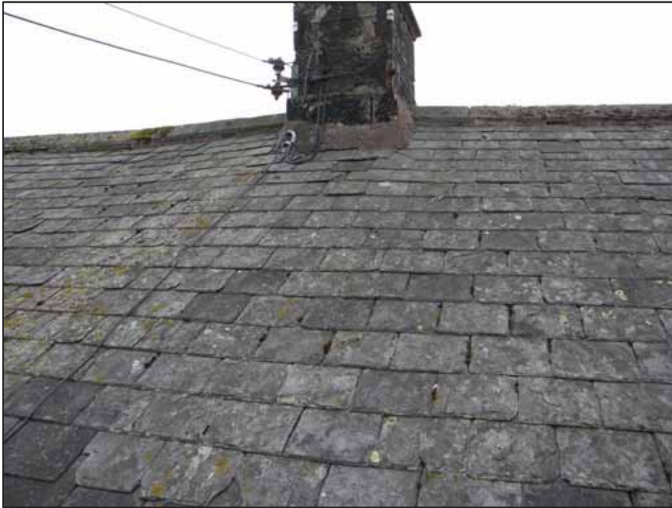
Figure 8. Roof to the rear.
