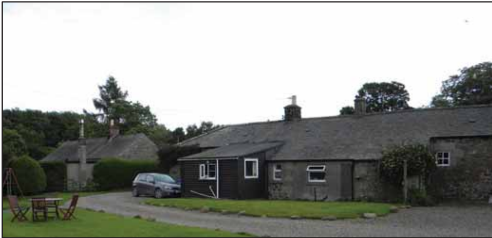
Figure 4. View from rear showing existing extension.
