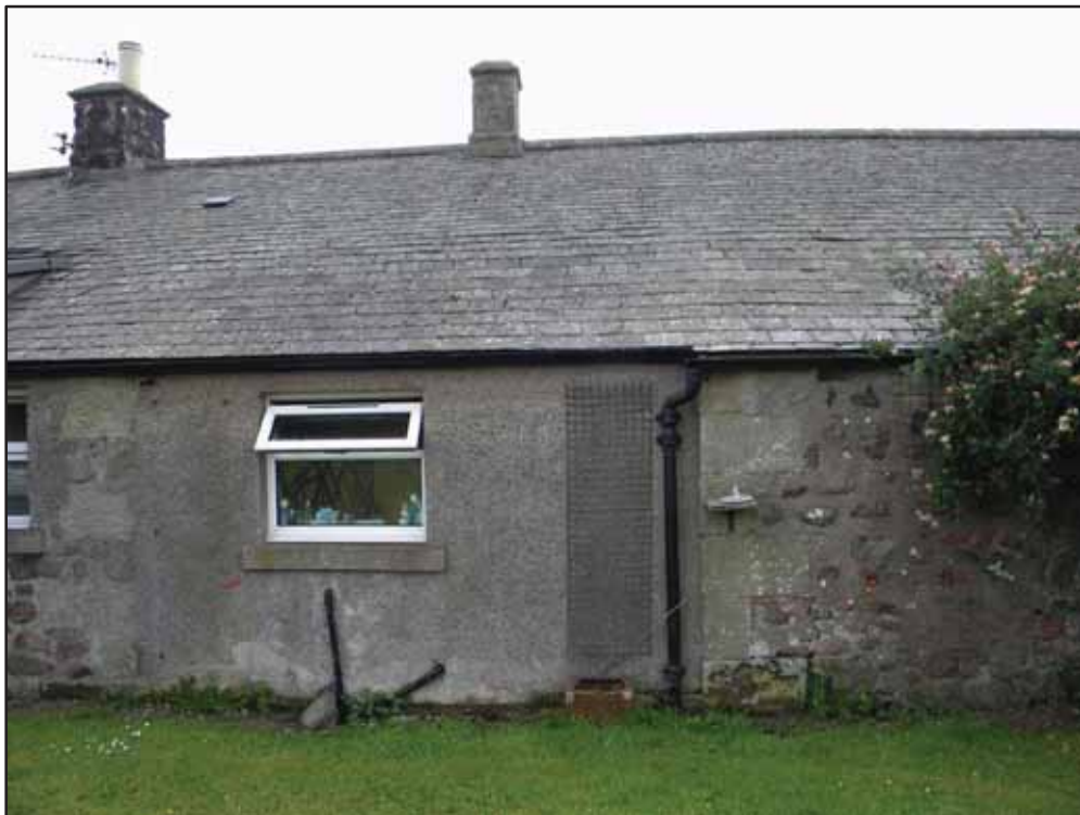
Figure 7. Rear wall (to be extended)
