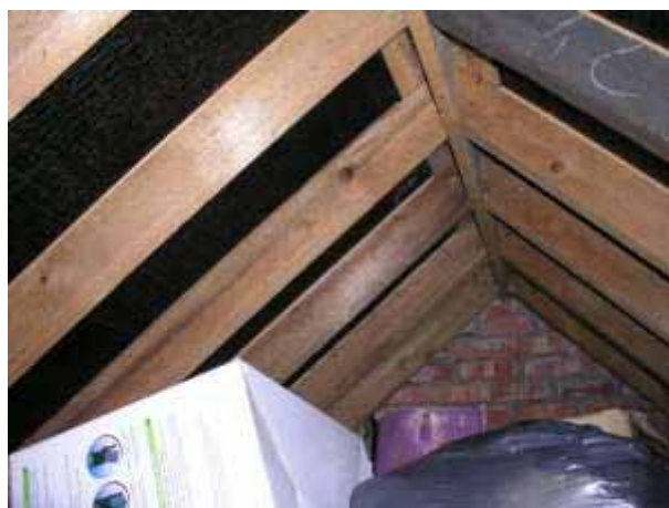
Interior of southern cottage loft with a felt sarking.
