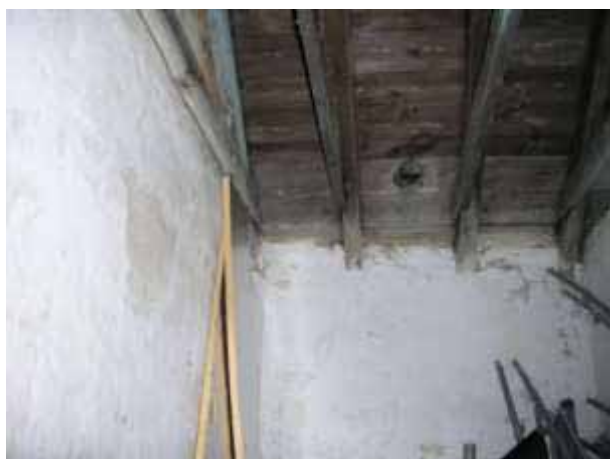
Interior of southern cottage loft with a felt sarking.
