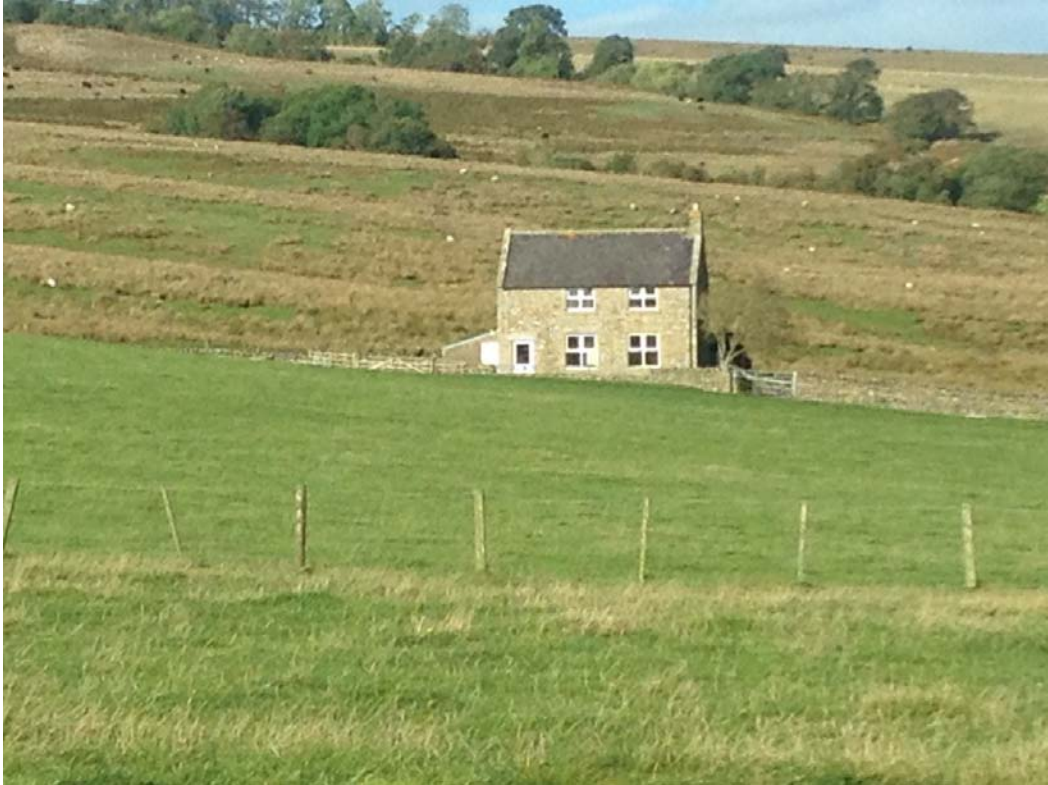
Existing cottage, photograph showing the southern elevation of the cottage. Proposed extension would be to the left hand side.
