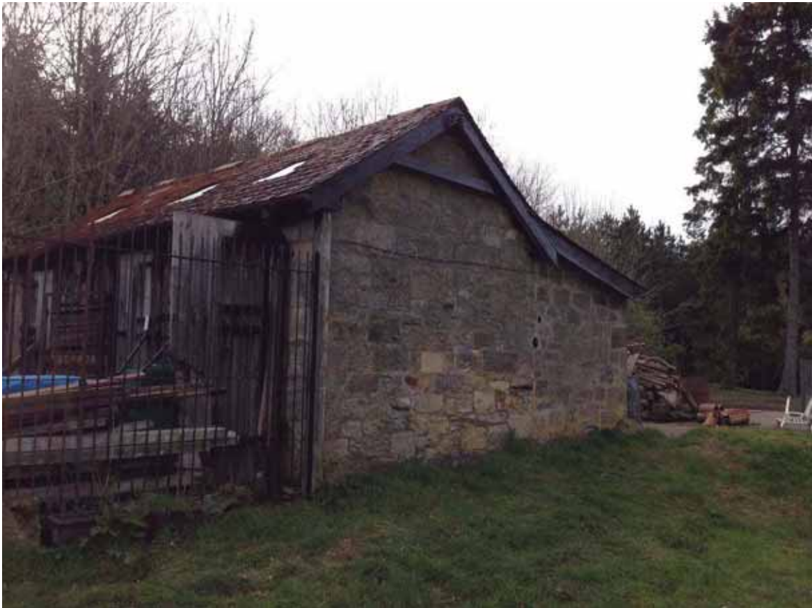
East elevation showing the remedial high level pointing to the lean-to section and the generally good condition of the stonework. Also the railings surrounding the kennel run to the south
