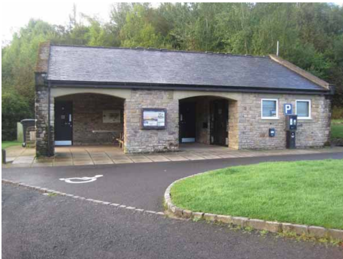
Front (north) elevation of the building, showing the covered outdoor space, which is to be modified to form the internal visitor centre/café area
