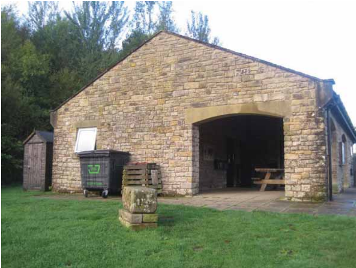
Side (east) elevation of the building, which is to be extended – the extension to the south elevation would be tucked away to the rear behind the shed to the left of the picture
