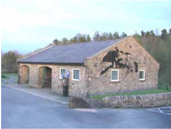
The building from the southeast.
