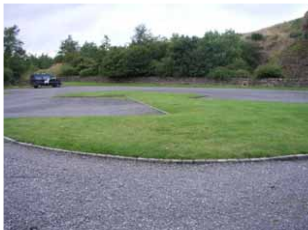
Looking along the east aspect of the building.
