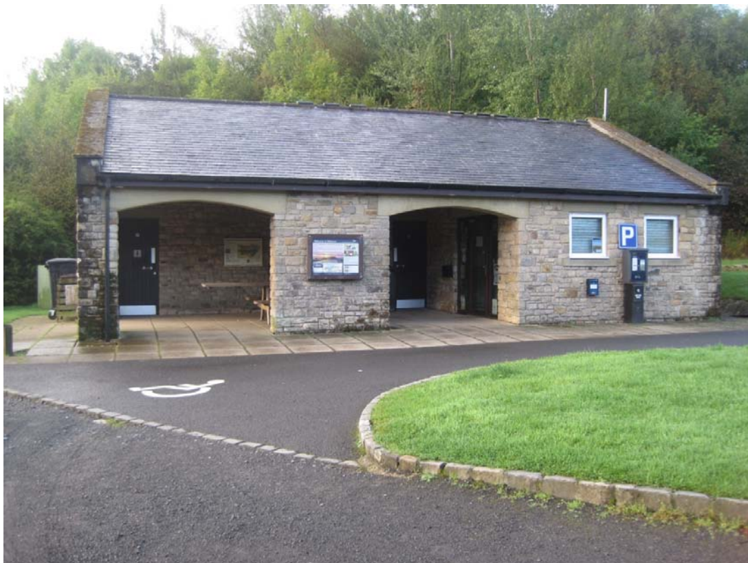
Front (north) elevation of the building as existing
