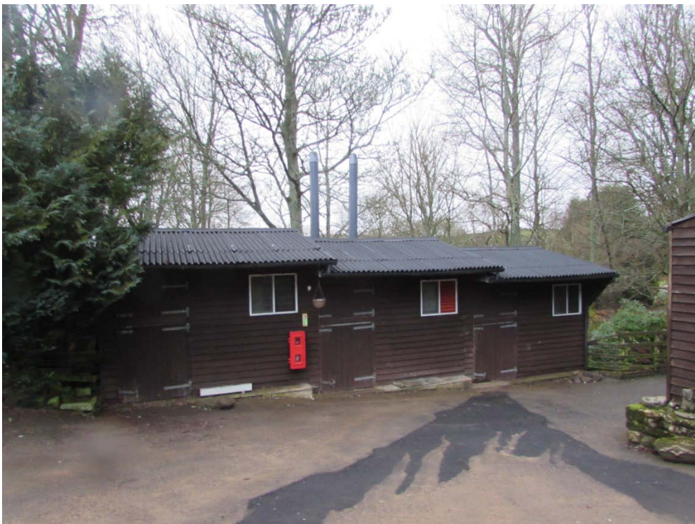
Front of stable building (with flues installed)
