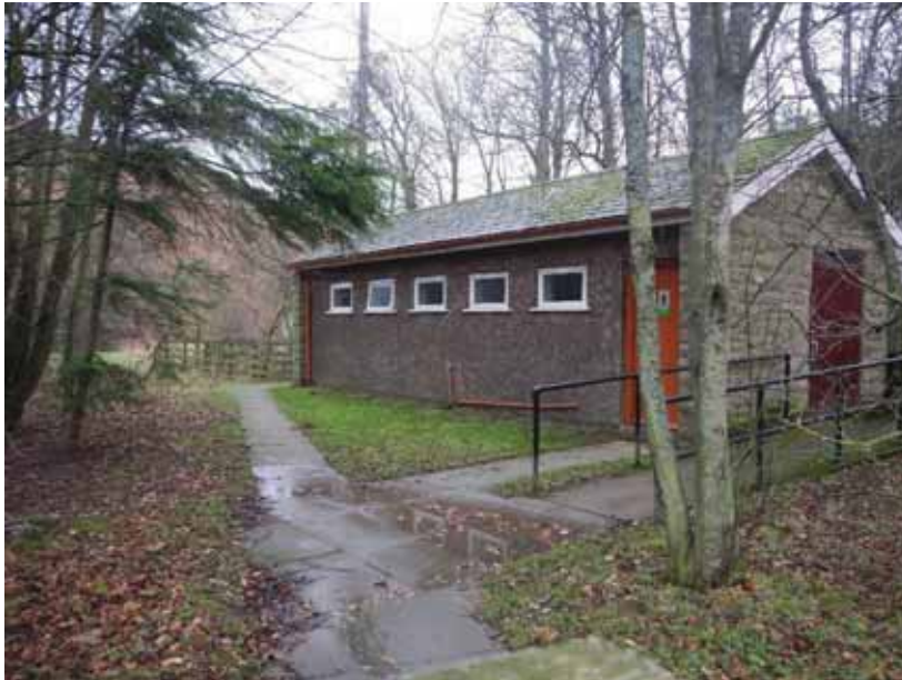
Photograph 1: The Bulby's Wood Toilet Block
