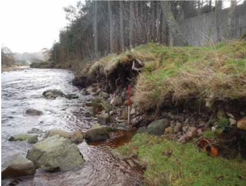
Photograph 5: Eroding bank to the north of the toilet block
