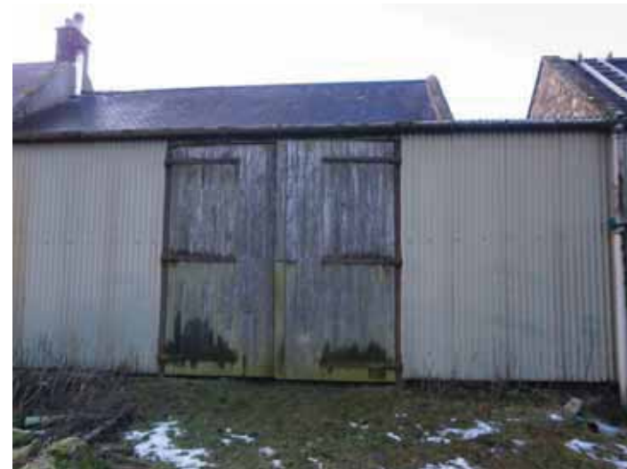
Existing Storage Outbuilding
