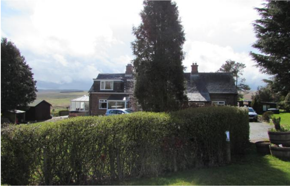
Front elevation of application site and adjoining dwelling, as seen from road verge adjacent to A68. Existing conservatory is visible to the left hand elevation of the pair of properties.
