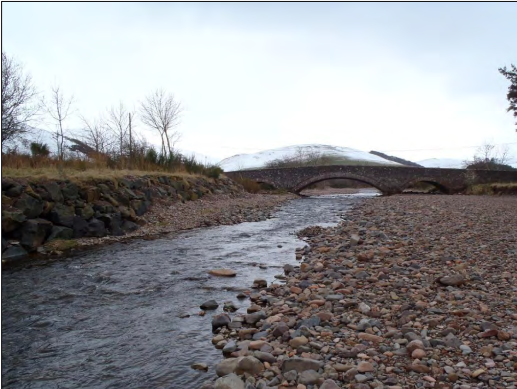
Figure 2.8. Looking upstream towards Westnewton Bridge showing straightened channel and bank protection on left of picture.
