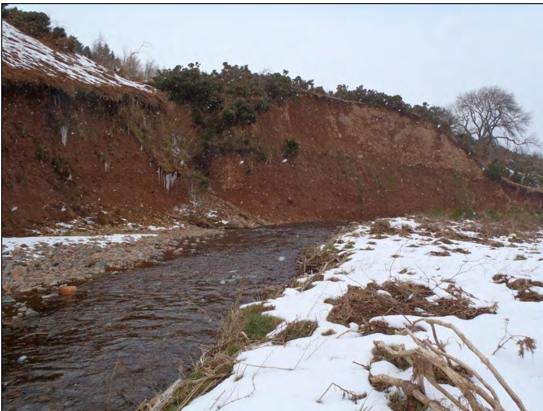
Figure 2.6. Terrace erosion in the central part of the reach.
