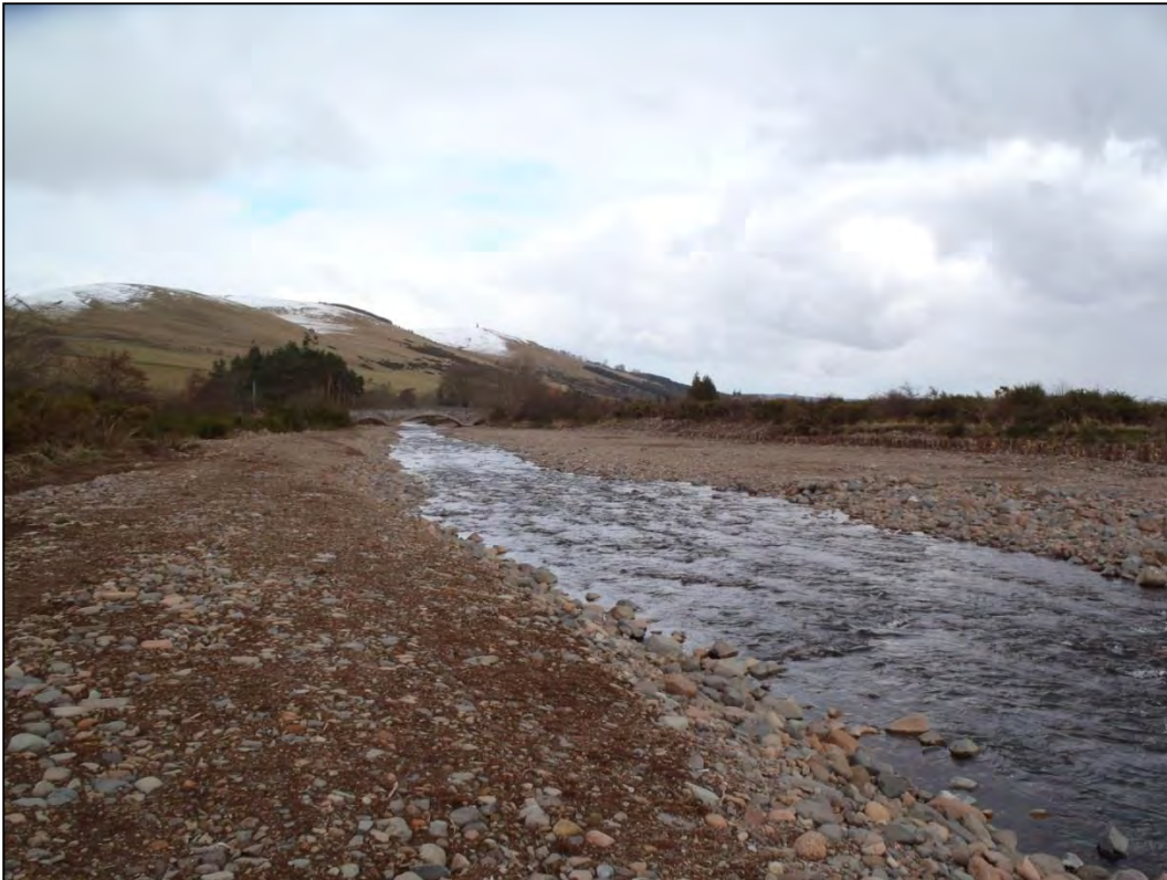
Figure 2.7. Straightened/ dredged channel upstream of Westnewton Bridge, showing embankment and bank protection on right.
