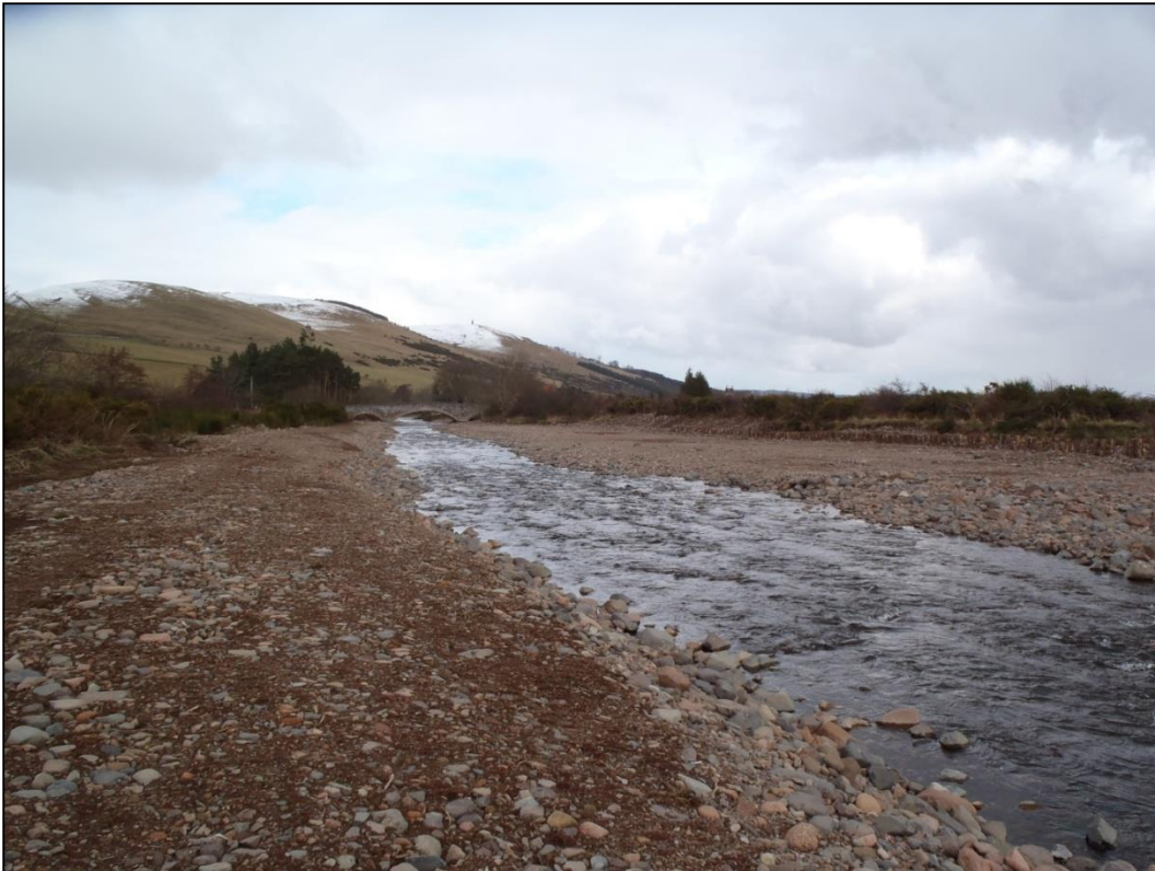
Figure 2.7. Straightened/ dredged channel upstream of Westnewton Bridge, showing embankment and bank protection on right.
