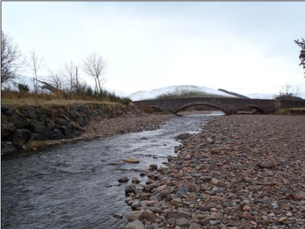
Figure 2.8. Looking upstream towards Westnewton Bridge showing straightened channel and bank protection on left of picture.
