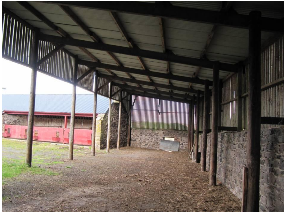
Photo 10. Traditional store barn (building 2c), viewed internally from the south-west.
