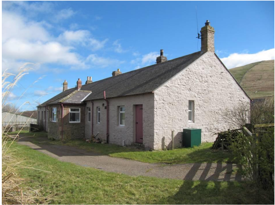
Photo 1. Bungalow (building 1), viewed from the south-west.
