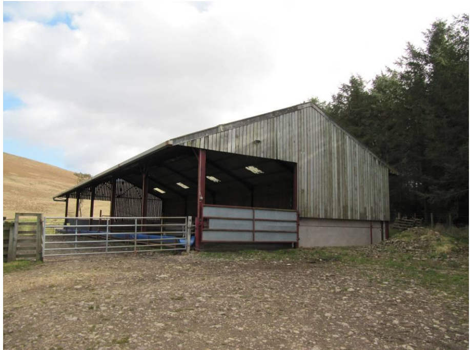
Photo 13. Modern steel-framed barn (building 3), viewed from the north-west.
