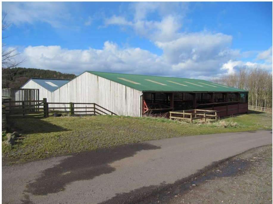
Photo 14. Modern steel-framed barn (building 4), viewed from the south.
