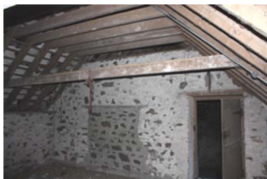
Figure 4 – Internal view of southern upper storey of the barn
