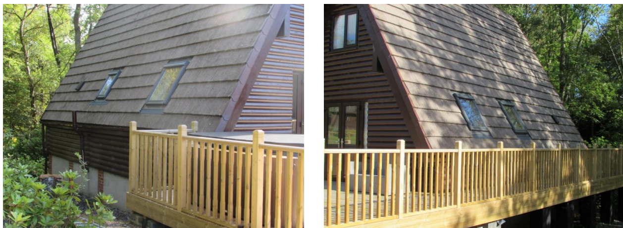
View of side elevations of Lodge 14, showing 4no. rooflights for which retrospective permission is sought
