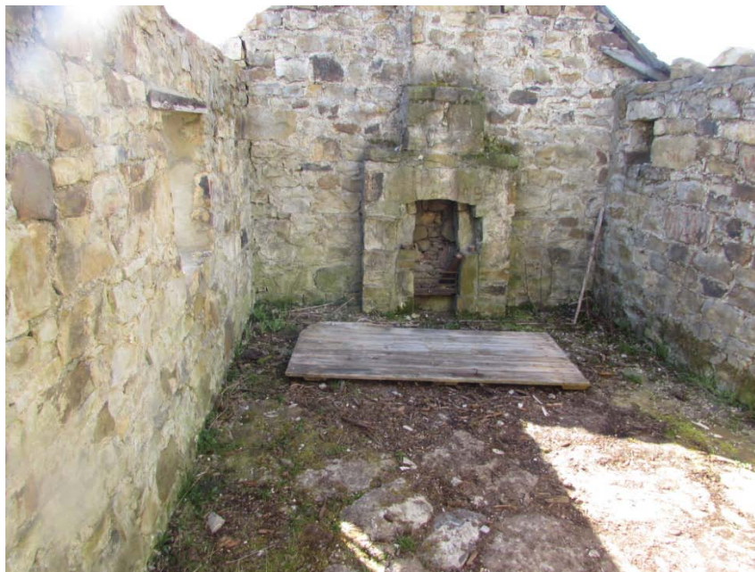
Existing interior of the bothy
