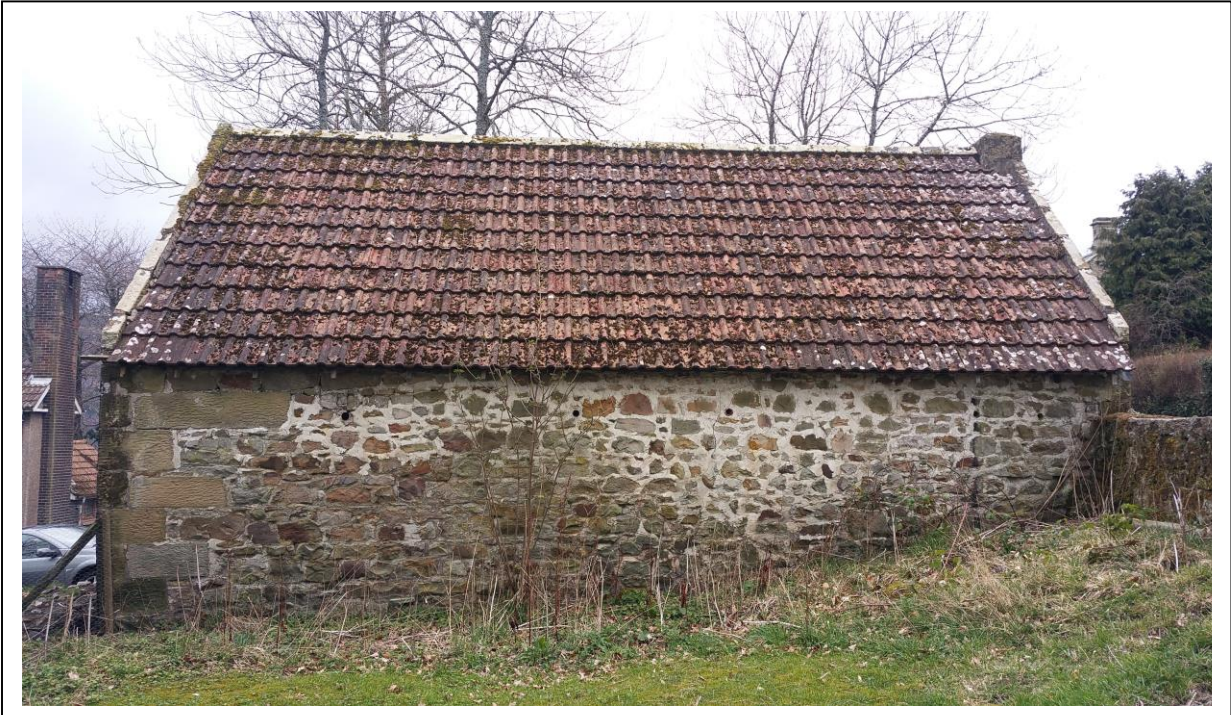
Eastern elevation showing repointing
