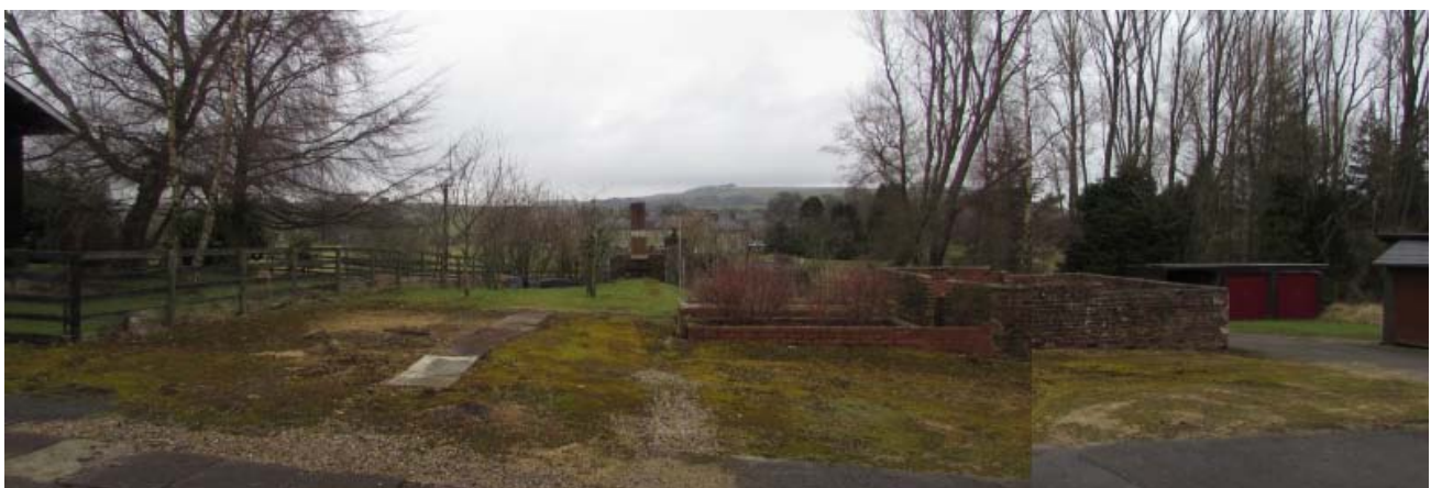
Photomontage of view north towards site of proposed compound; brick foundations to be removed
