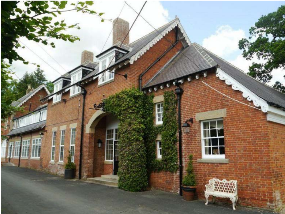
View facing north west towards front elevation of The Coach House. Dovecote Cottage visible to far left (east)
