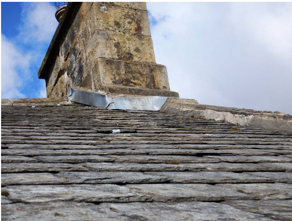
Water tabling and flashing back West end
