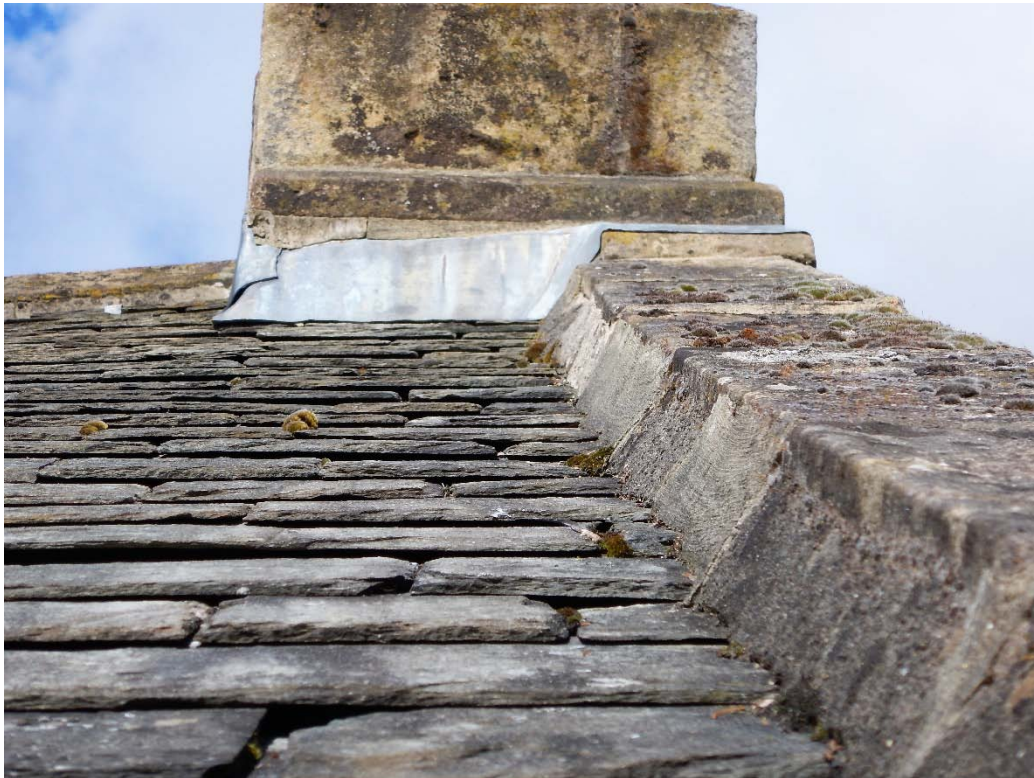
Water tabling and ridge rear elevation
