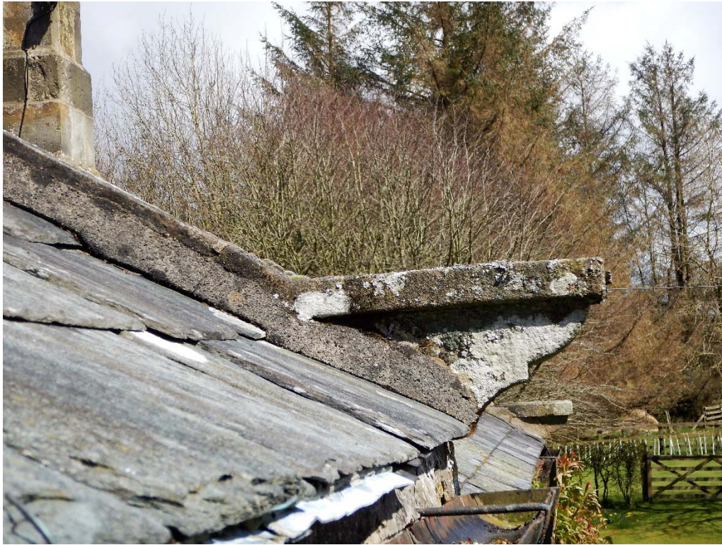
Water tabling fillet Front Roof East End
