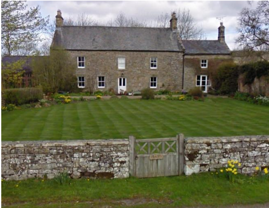
View facing north towards front elevation of property
