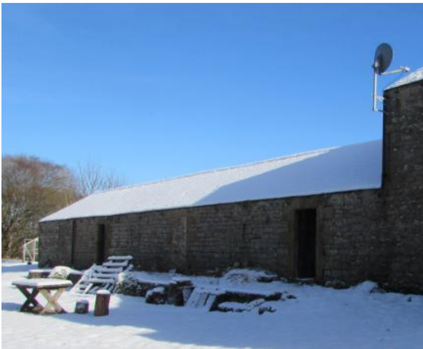
Left: North west facing elevation of building; blocked up doorway visible to centre (lighter colour stone)
