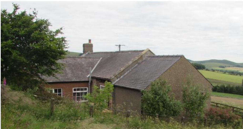
View facing north towards property showing partly-pebbledash rendered side extension and brick extension to rear (west)
