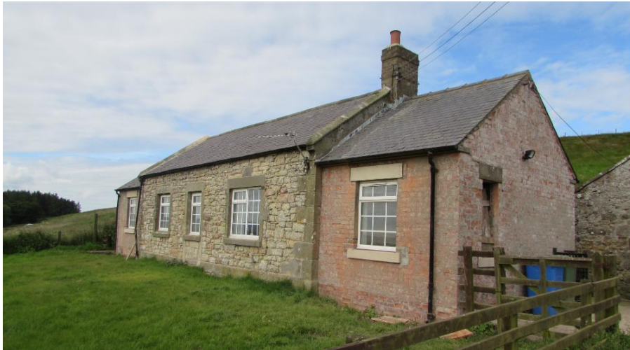
East face (front) of property showing brick 'wing' extensions to north and south (formerly pebbledashed)
