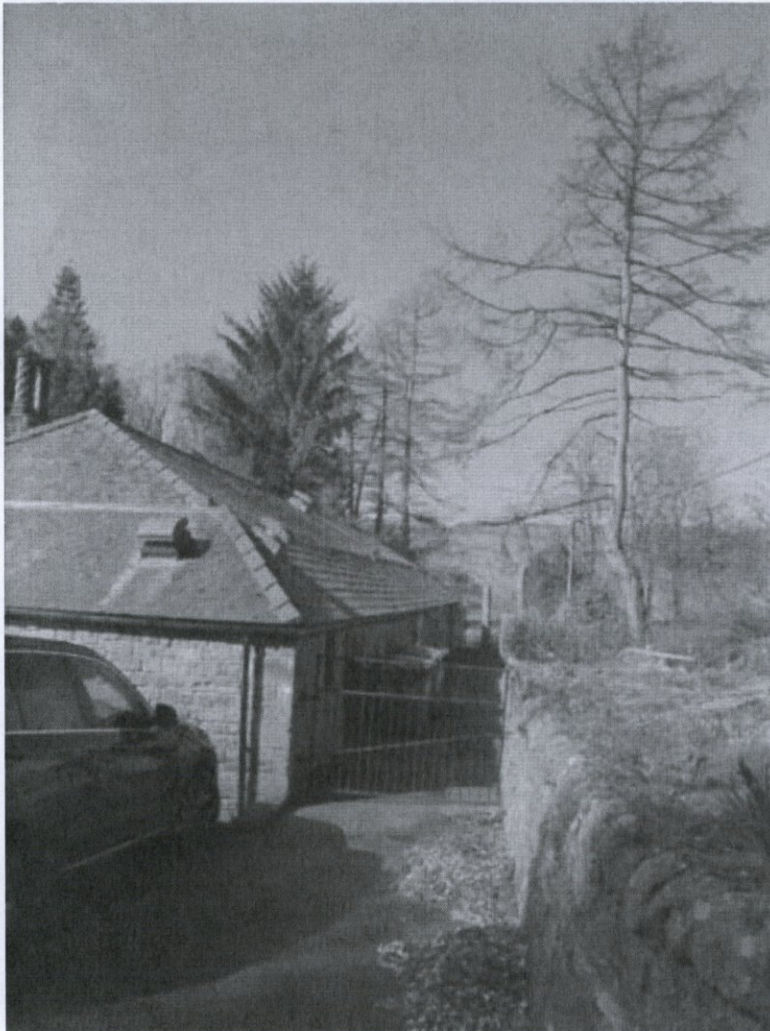
Photograph 3 Northern elevation of Building A1, where proposed extension will be carried out.
