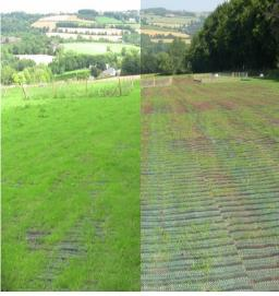
the new car parking area was used for the first time just a month afterwards. By retaining and reinforcing the grass the client was able to make use of the area in its first summer season. Avoiding excavations and lengthy waiting times for grass to establish was key to the success of this installation.
