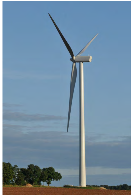
Wind Turbine 130 m to tip - St Seine Wind Farm, France
