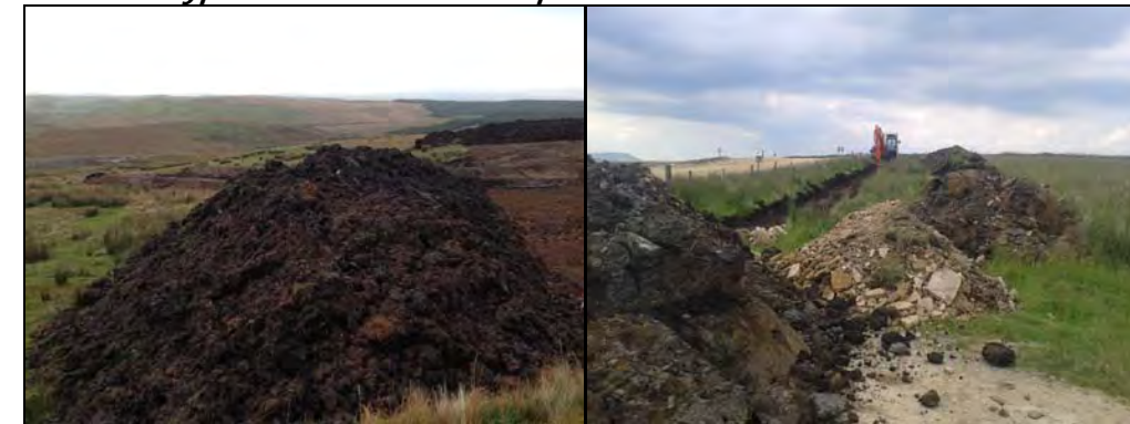
Plate 14: Typical overburden stockpile measures
