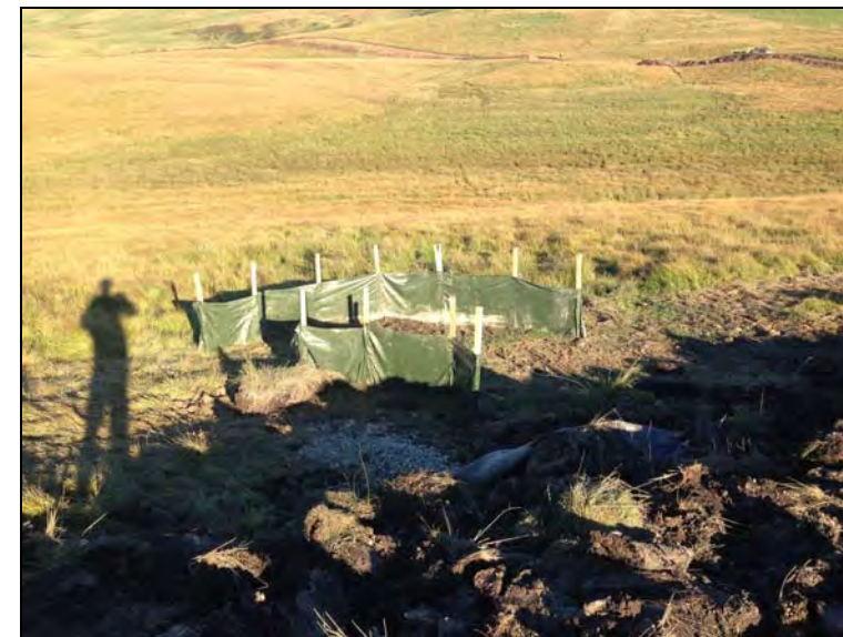
Plate 2: Typical silt traps
