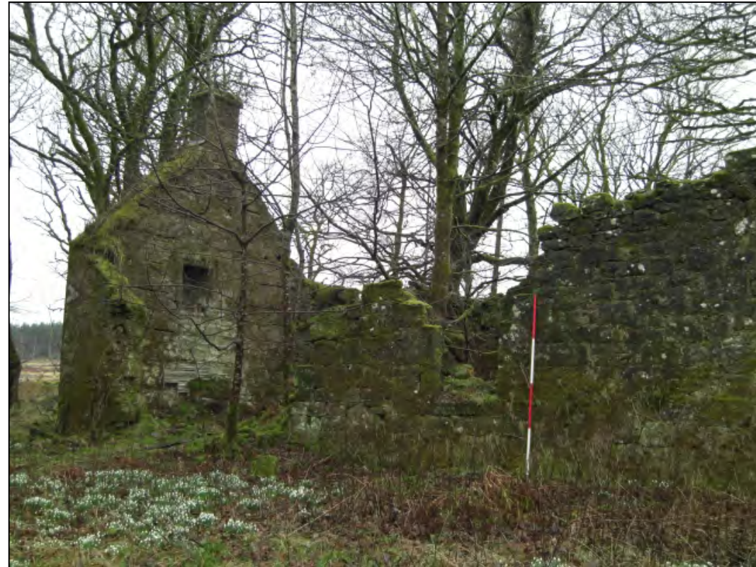
Plate 7a – Detail of the ruins of Westshiels Farmstead (Site 112)
