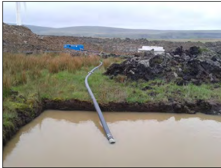
Plate 6: Typical 'Siltbuster' and settlement lagoon
