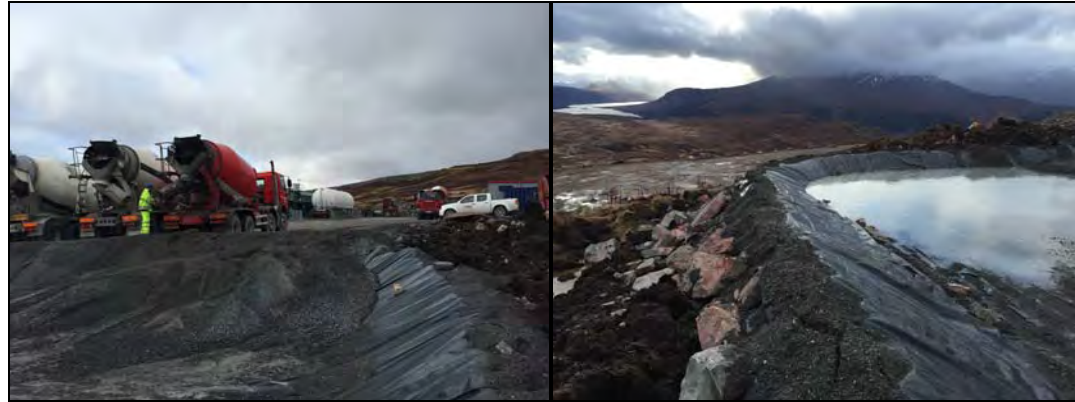
Plate 8: Typical concrete washout facility
