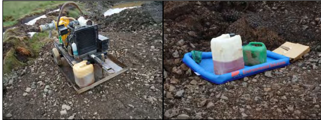
Plates 11 and 12: examples of drip trays and bunds
