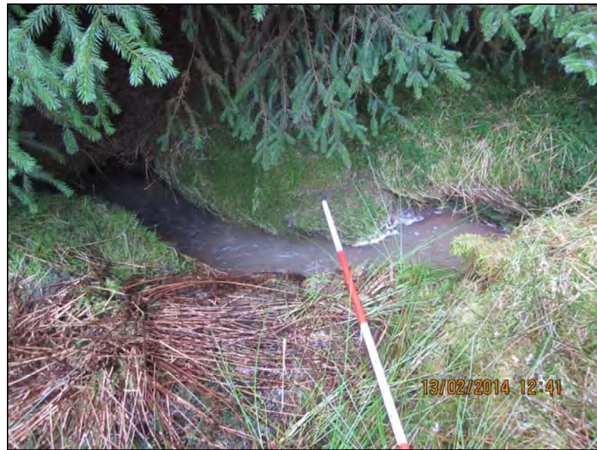
Crossing Location Upstream
