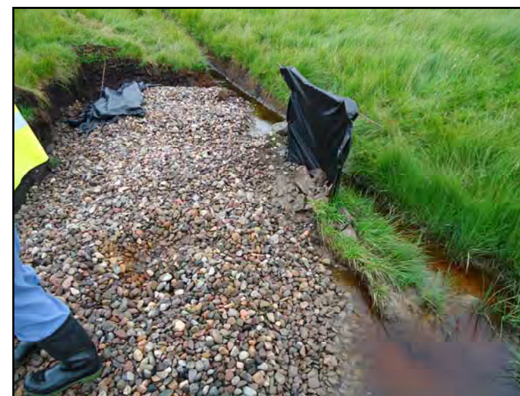
Plate 2: Typical silt traps
