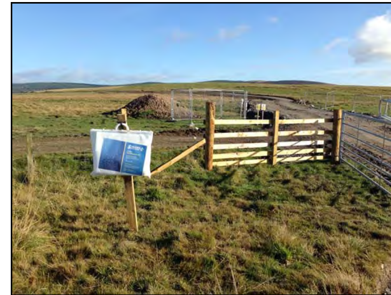
Plate 7: Spill Kits to be located across the Development
