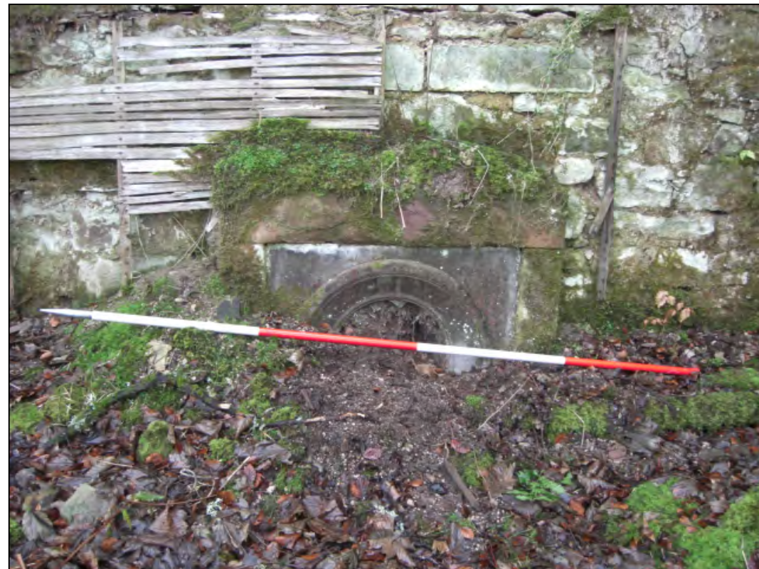
Plate 7b - Detail of the ruins of Westshiels Farmstead (Site 112)
