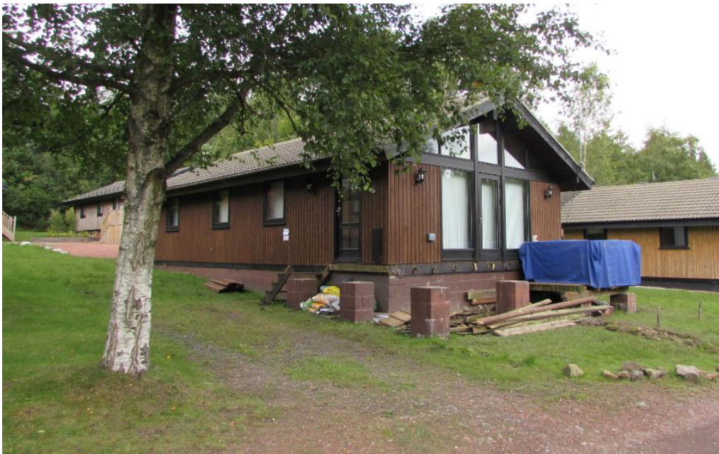
Lodge 6 with decking part-removed
