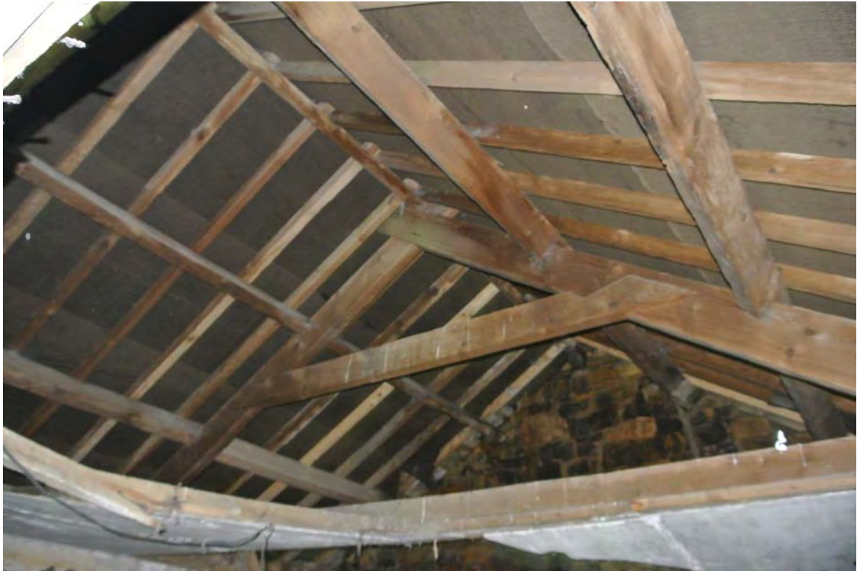
View of existing roof structure showing bitumen felt etc.
