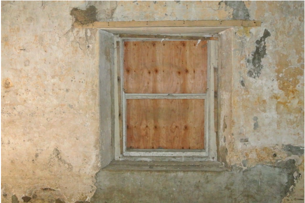
Existing sliding sash window to South elevation in Area 1
