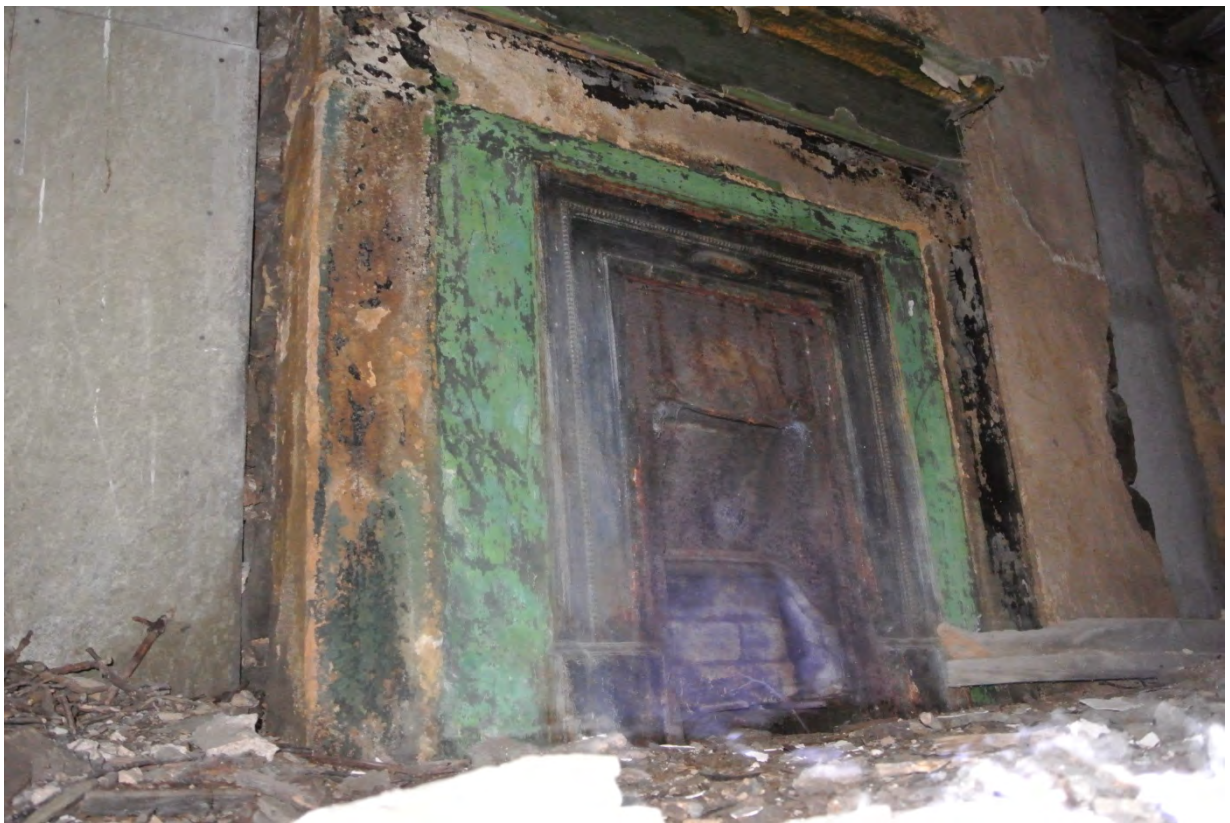
Detail of fireplace to West at first floor
