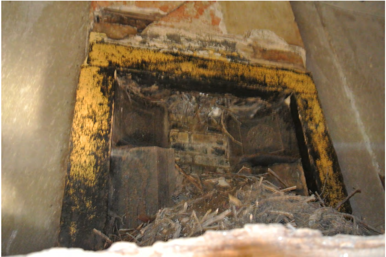
Detail of fireplace to East at first floor
