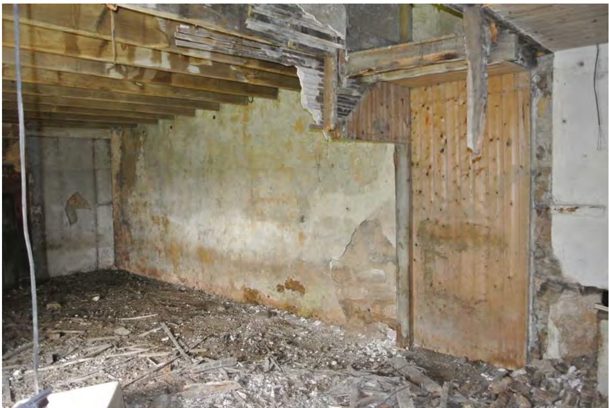
View of North wall at ground floor showing landing
