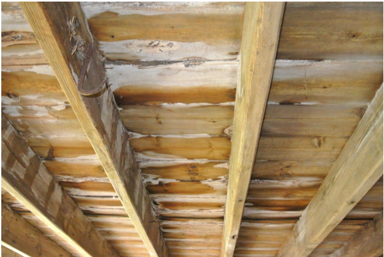
View of rotten floorboards in Area 2 and hooks to be reused
