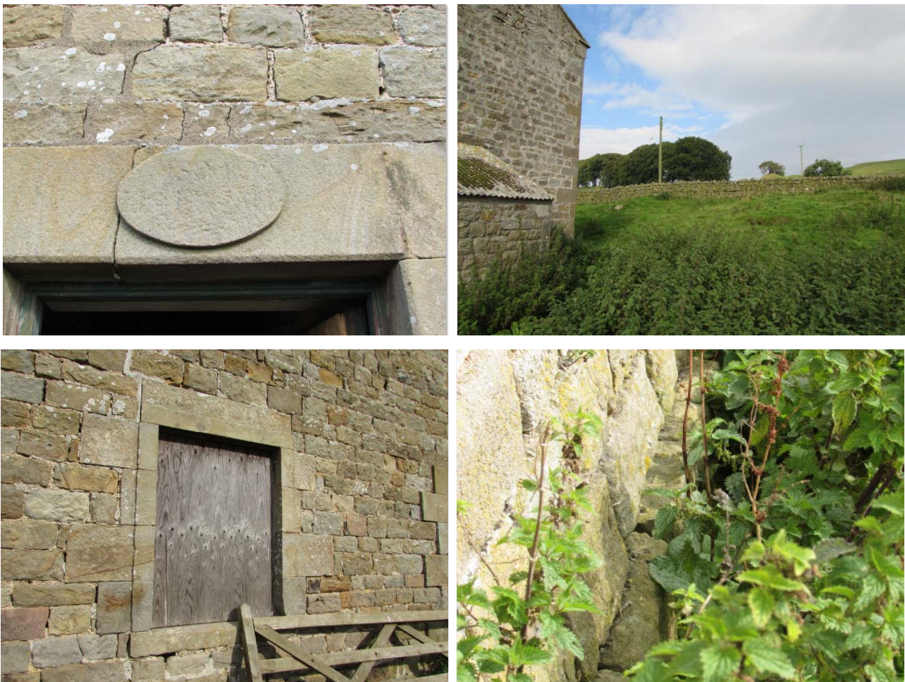
Fig. 4 (clockwise from top left): Oval datestone above entrance; alternating stone quoins to NE corner (stone lean-to visible); stone 'skirt' to foot of building; example of stone window surround
