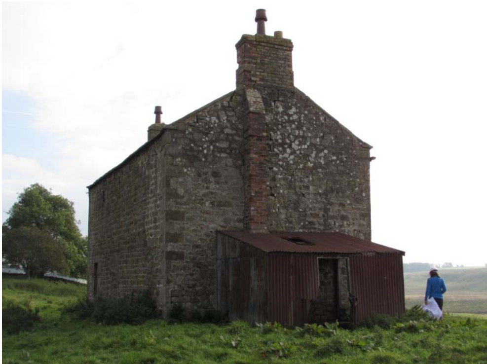
Fig. 5: View facing east towards existing corrugated steel extension
