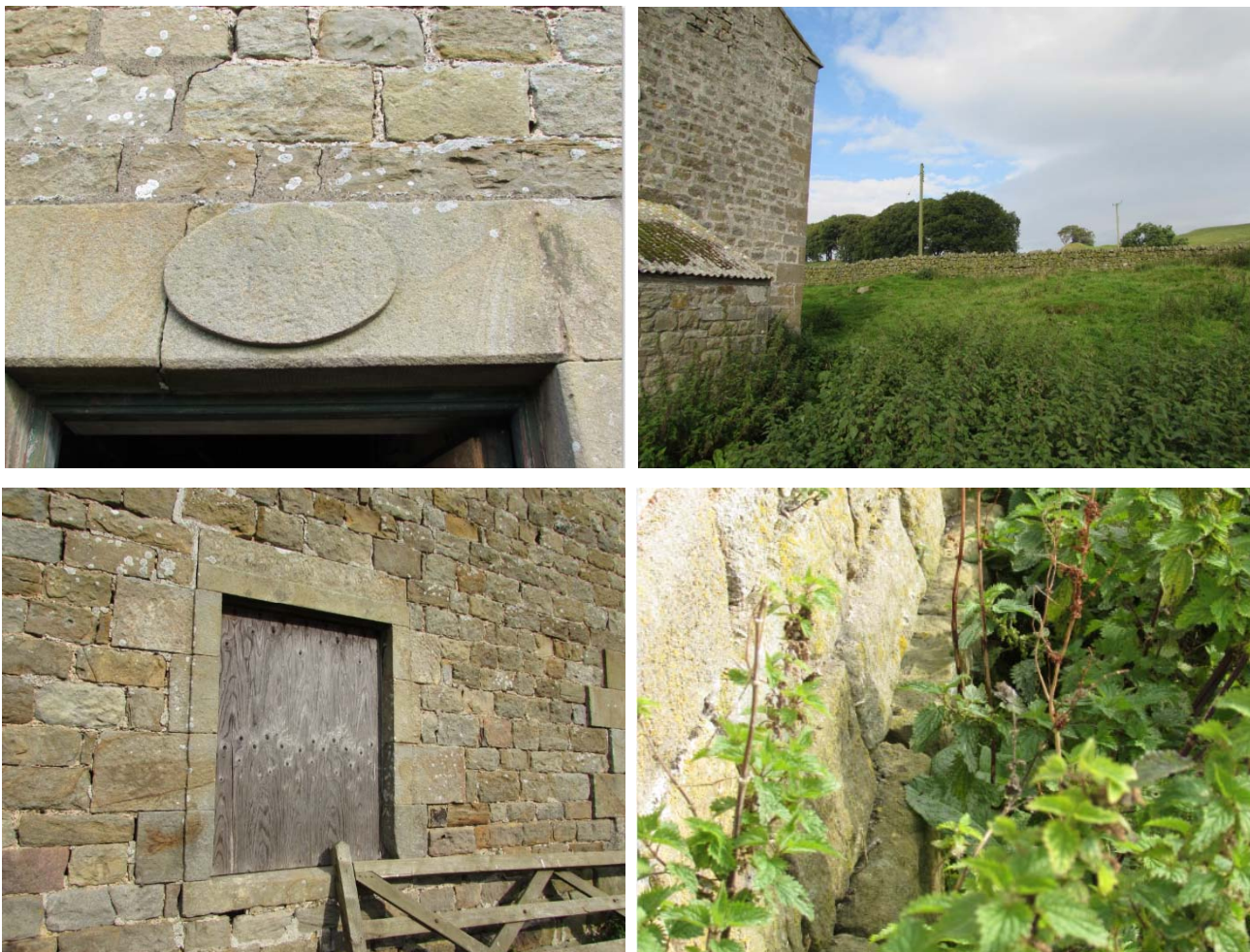
Fig. 4 (clockwise from top left): Oval datestone above entrance; alternating stone quoins to NE corner (stone lean-to visible); stone 'skirt' to foot of building; example of stone window surround
