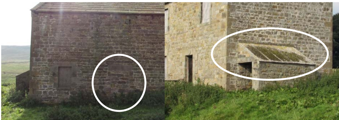
Fig. 10 (left): Location of blocked up doorway; (right): Roof of lean-to to be replaced
