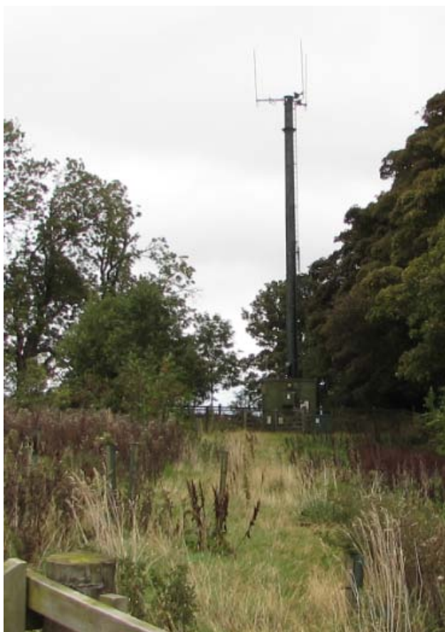
Left: View facing west towards application site
