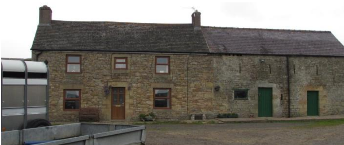
Front elevation of Greengate Well, facing towards yard
