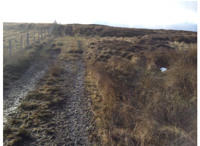
Photo 6: Close up of extensively rutted/eroding area mid-way up track route
