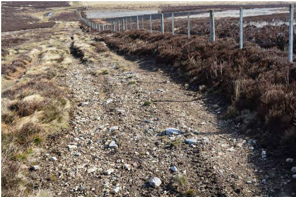
Photograph 3: Existing Track (deterioration)
