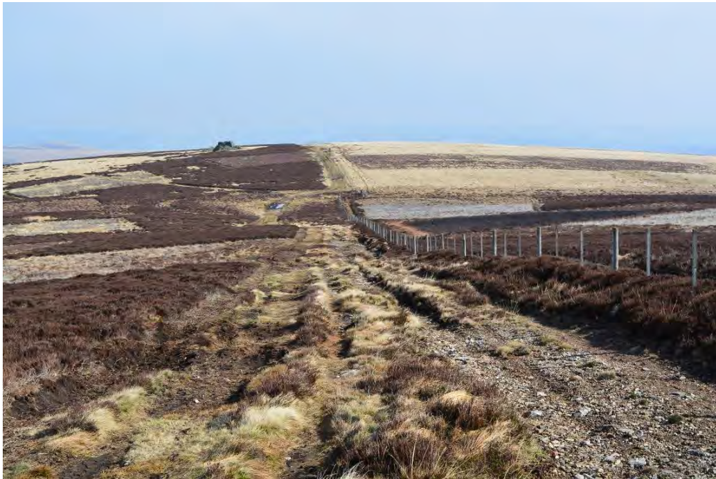
Photograph 2: Existing Track (widening)
