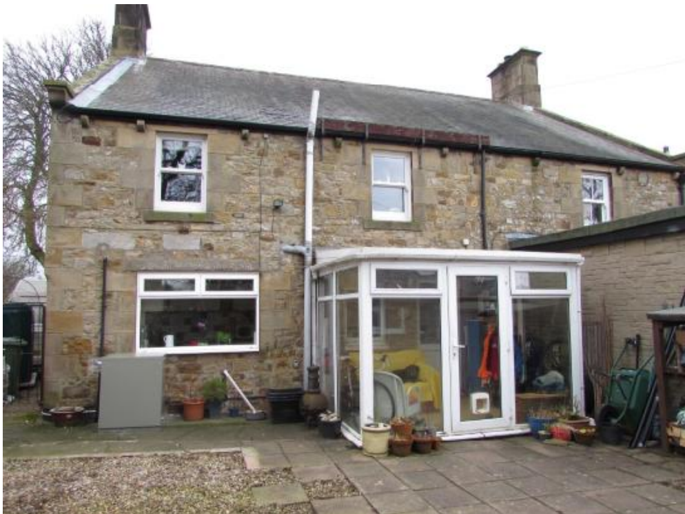
Existing rear (west-facing) elevation of property
