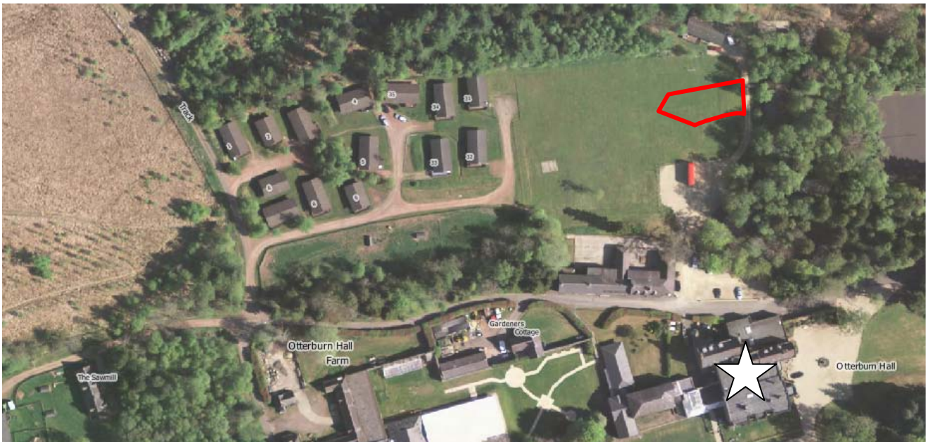
Aerial view of Otterburn Hall and 'top site'. Approximate position of site outlined in red. Otterburn Hall annotated with star. Partially-built chalets now covering formerly vacant land
