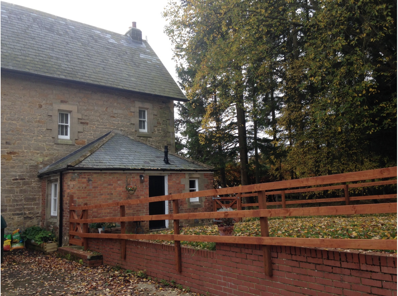
Photo 3: Fence following existing retaining wall of adjacent car park
