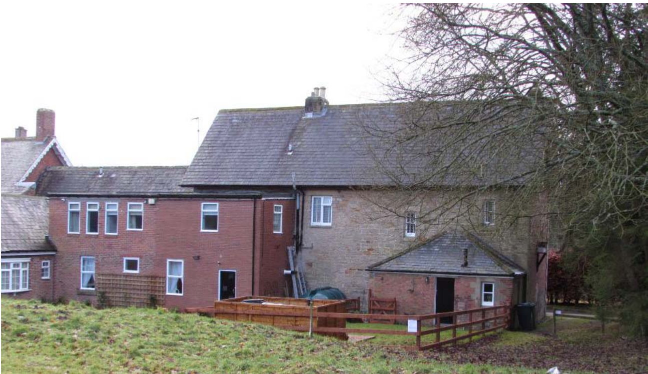
North-facing (rear) elevation of Dovecote Cottage
