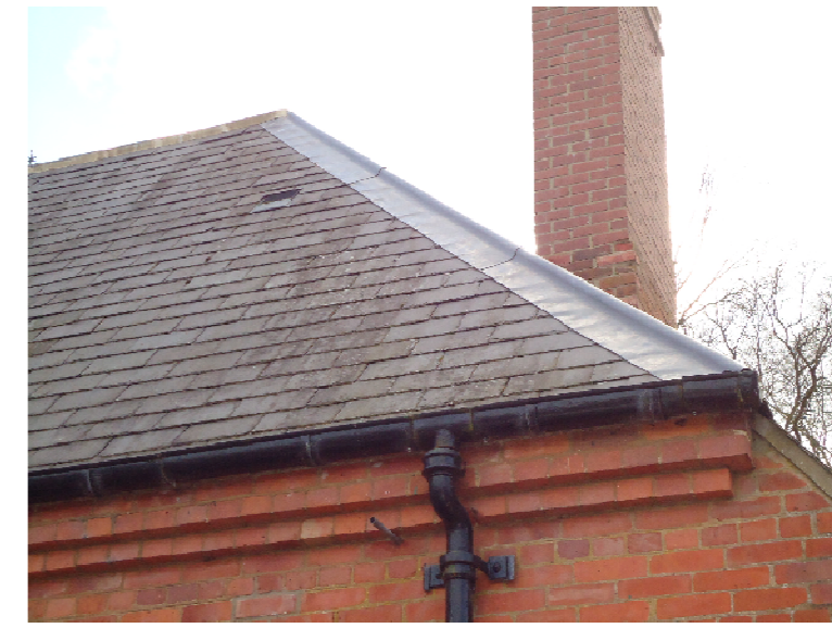
Code 4 Lead Hip Detail
