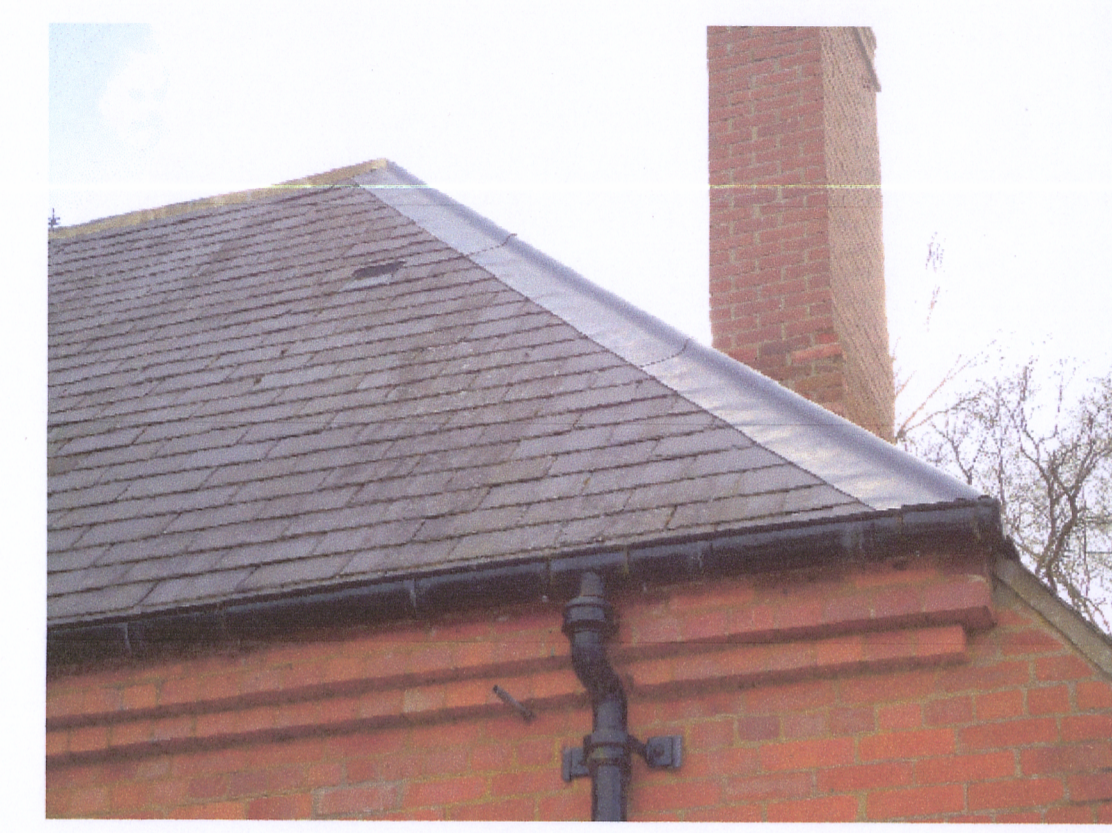
Code 4 Lead Hip Detail
