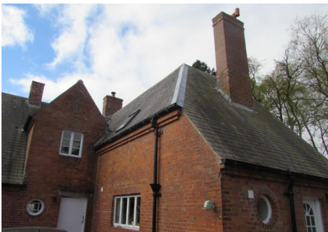
Left: Roof light window to north eastern side
