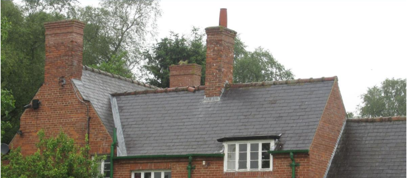
2013 photograph showing former roof tiles and overall condition
