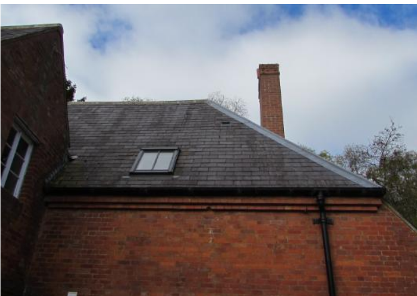
Images of rooflight window installed to north eastern roofslope
