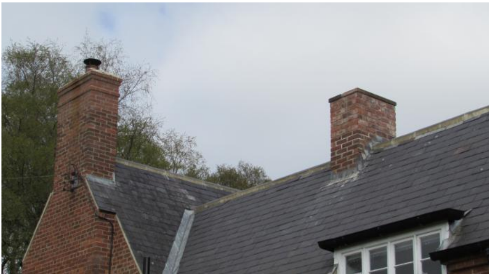
Photograph taken 09.05.2017 showing present roof condition
