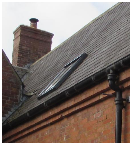
Images of rooflight window installed to north eastern roofslope
