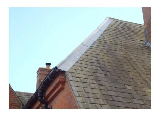
Photograph of the property (left) taken around 2014 showing the significant amount of vegetation growth within the roof gutters. Photograph right showing the new code 4 lead roof hip.
