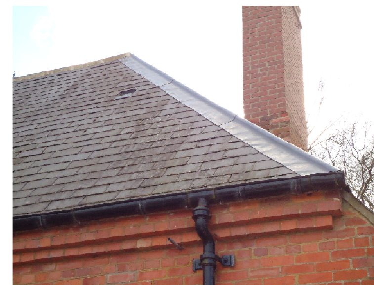
Code 4 Lead Hip Detail
